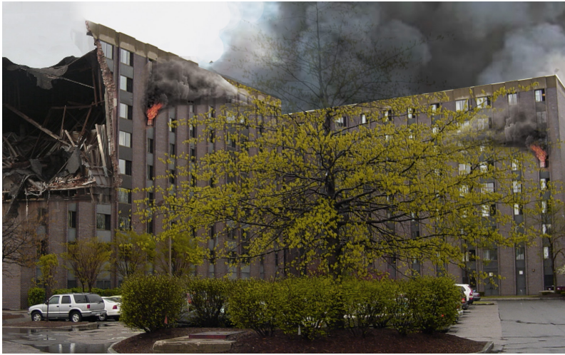
"YOU GUYS NEVER SAID ANYTHING ABOUT CONTROLLED DEMOLITION!"
